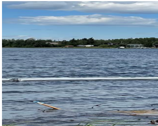
Single semi-permeable curtain in use along a lake shoreline construction site.
